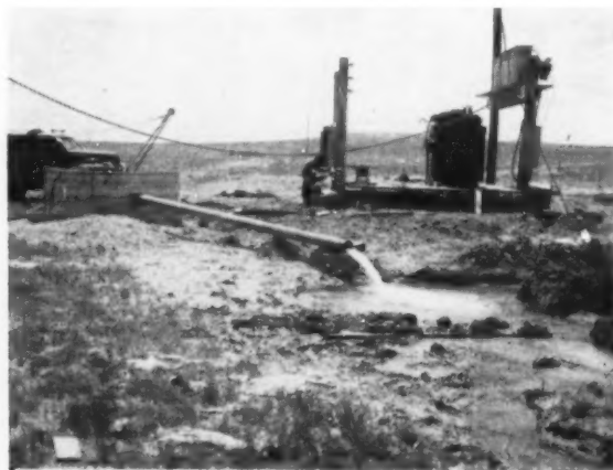
WELLS containing submersible pumps have lowered the water table by pumping over 6,500 gallons of water a minute.
